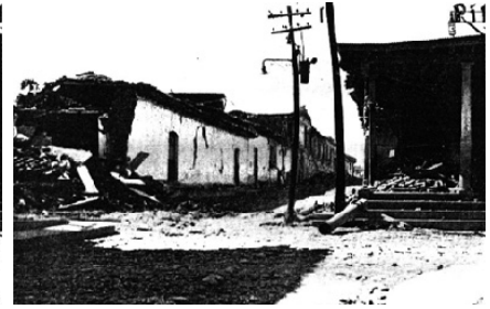
Figure 6C: Damage to an adobe church in the 1999 Apastepeque earthquake
