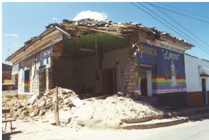
Figure 6G: The San Jose church, Cojutepeque, damaged in the 13 February 2001 earthquake
