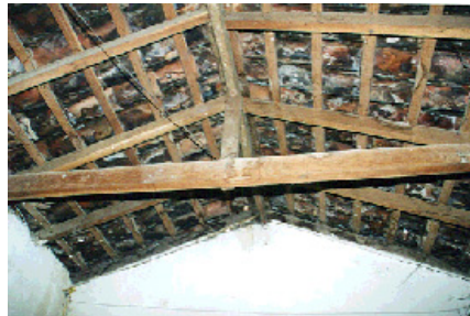
Figure 4A: Critical Structural Details: An illustration of wood beams supporting clay tiles and roof-walls connections
