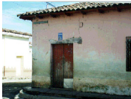
Figure 5B: Deficient bedding of lintels
