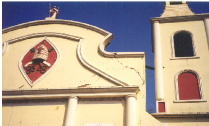
Figure 6D: Wall damage (corner separation) in the 1999 Apastepeque earthquake
