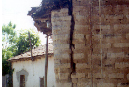
Figure 6E: Damage in the town of Juayua due to the January 13, 2001 earthquake
