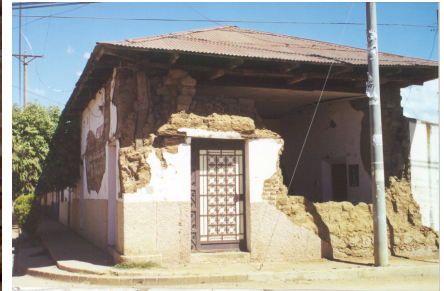
Figure 6F: Damage in the city of Cojutepeque due to the February 13, 2001 earthquake
