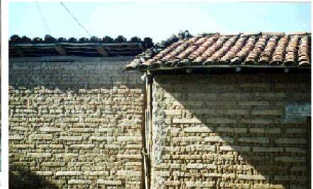
Figure 4B: Wall connections
