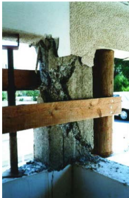
Figure 6E: Shearing of concrete and buckling of
