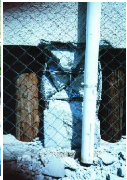
Figure 6F: Torsional shearing and buckling of
