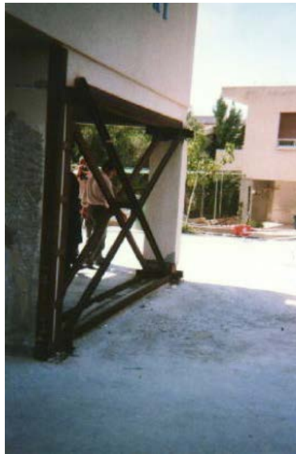
Figure 7E: Infillings. a) Into opening, b) Into frame, c) Steel bracing, d) Panel with opening
