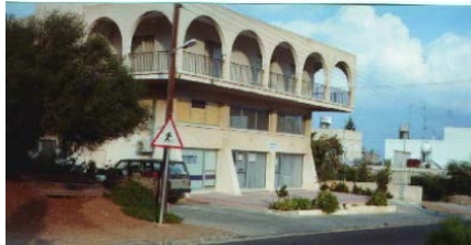
Figure 5J: Weak columns, incomplete beam-grid and a heavy-rigid parapet wall of the additional constructed top story
