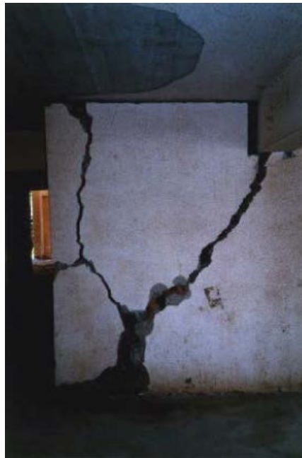
Figure 6B: Diagonal shearing of an infill wall
