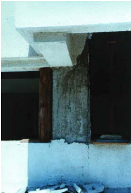
Figure 6J: Support failure
