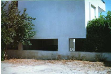
Figure 5G: Excessive length of a cantilever canopy
