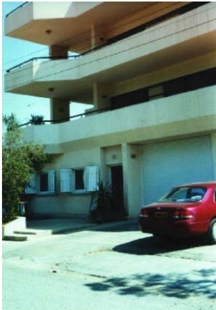
Figure 5I: Heavy concentrated loads are transferred to a thin balcony slab
