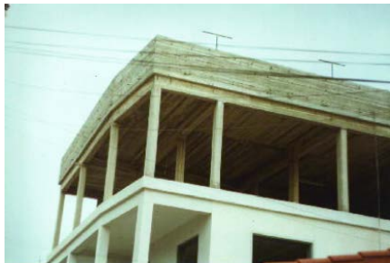
Figure 6A: A Photograph Illustrating Typical Earthquake Damage. Shearing failure of a partition
