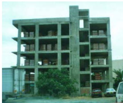
Figure 5C: Non symmetrical location of stairwell
