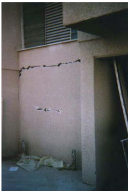
Figure 6D: Shearing failure of a short column
