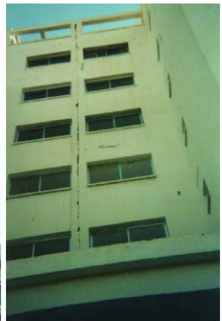
Figure 5D: Inadequate seismic joint
