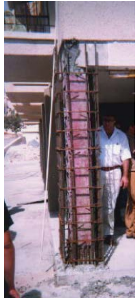
Figure 7C: Confining of concrete by spiral wire
