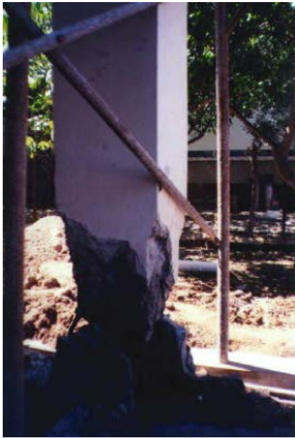
Figure 6G: Shearing and buckling at the bottom of a column
