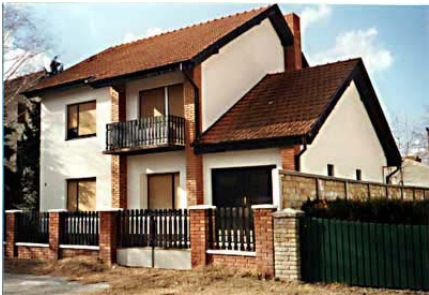
Figure 1A: Typical Building
