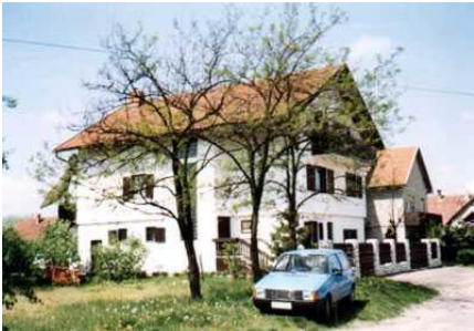
Figure 1B: Typical building
