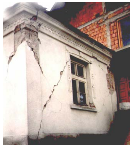
Figure 6: Damage to masonry buildings in the 1998 Mionica earthquake
