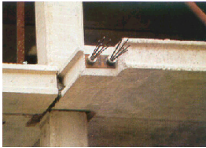
Figure 4B: Details of a typical post-tensional slab-column connection
