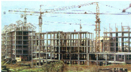
Figure 1B: IMS Buildings under construction
