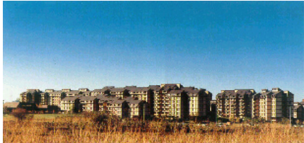
Figure 1C: A block of buildings constructed using IMS technology
