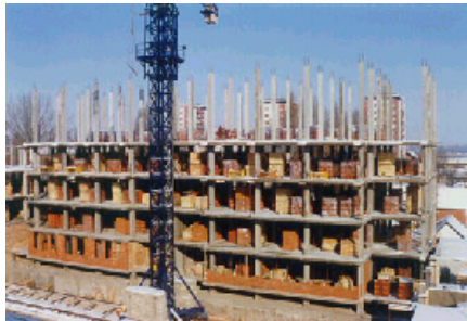
Figure 8: An Illustration of column erection
