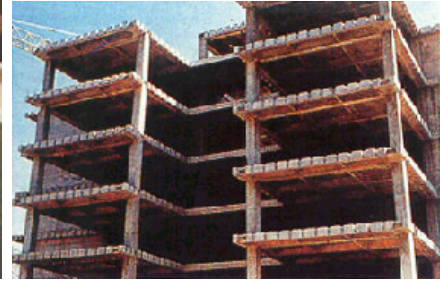
Figure 4C: Details of an IMS building under construction showing cantilevered balcony slabs
