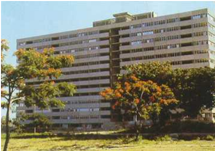
Figure 1A: Typical building
