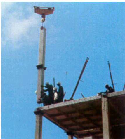
Figure 9: A high-rise building under construction
