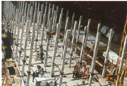
Figure 6: A medium-rise residential building under construction
