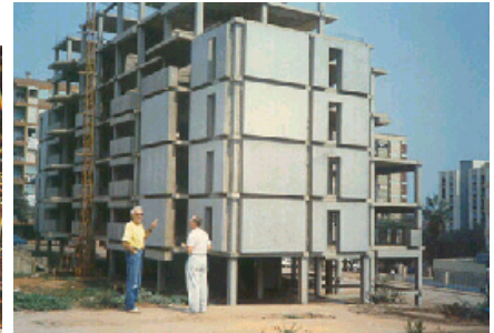
Figure 7: A building under construction, showing columns at the top floor erected in the vertical position
