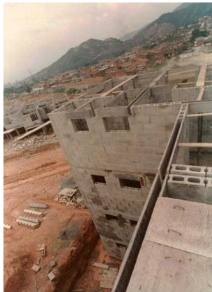
Figure 4B: Critical Structural Details - Modern buildings Built with Continuous R/C Bond Beams
