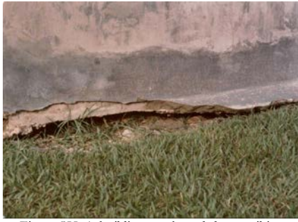
Figure 5H: A building weakened due to tilting induced by a pre-earthquake foundation settlement (separation between the two buildings was 100 mm at ground level but 0 mm at the top). Such buildings are likely to suffer more extensively earthquake damage
