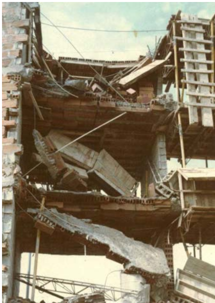
Figure 5E: Seismic Deficiencies - An Example of a Building Collapse Caused by Gravity Loads Only (buildings with such weaknesses have very little chance to survive earthquake effects)
