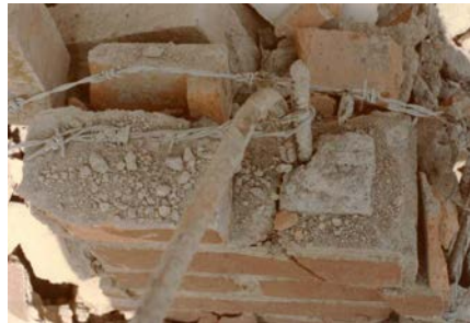
Figure 5F: Seismic Deficiencies - Poor Quality of Materials (mortar and grout); Inadequate Vertical and Horizontal Reinforcement
