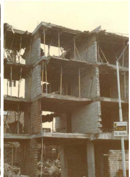
Figure 5D: Vertical Stiffness Discontinuity - Walls Interrupted at the First Story and Replaced with Columns
