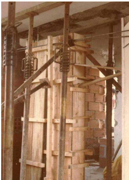
Figure 7A: Seismic Strengthening Techniques-Installation of New Concrete Tie Columns
