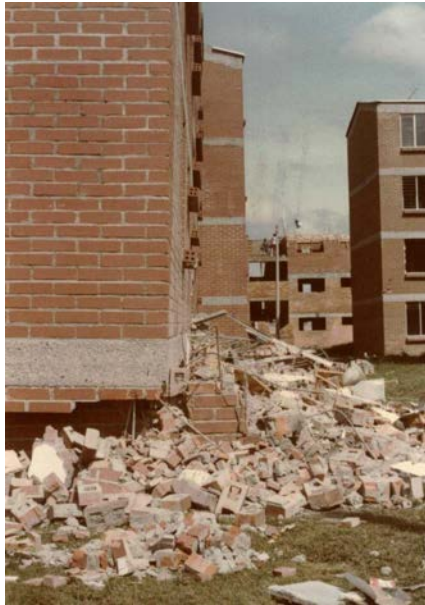
Figure 6C: Typical Earthquake Damage - Lateral Movement of the Collapsed Building Relative to the Foundations
