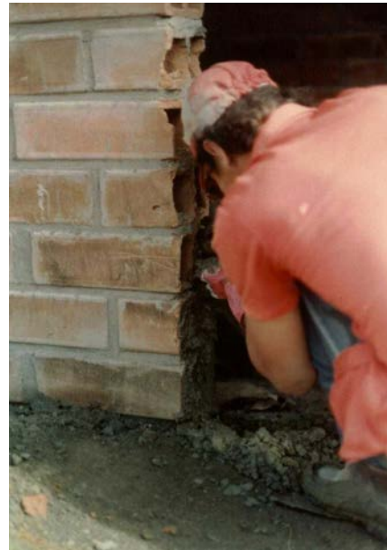
Figure 7B: Seismic Strengthening Techniques - Installation of New Concrete Tie Column
