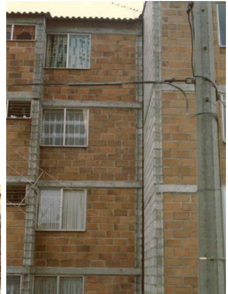
Figure 5G: A building weakened due to tilting induced by a pre-earthquake foundation settlement (separation between the two buildings was 100 mm at ground level but 0 mm at the top). Such buildings are likely to suffer more extensive earthquake damage
