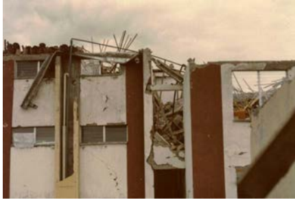
Figure 5B: Seismic Deficiencies - Discontinuous R/C Bond Beams
