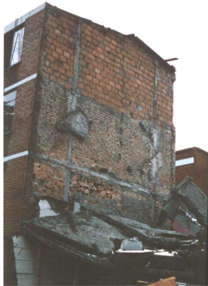
Figure 6F: Typical Earthquake Damage Illustrating Two Similar Confined Masonry Buildings (note that the building on the right-hand side collapsed while the one on the left remained standing)
