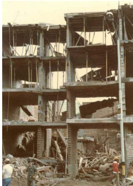
Figure 5C: Poor construction practice - unreinforced masonry walls and the absence of cross walls (note that both clay bricks and concrete blocks were used for the wall construction)
