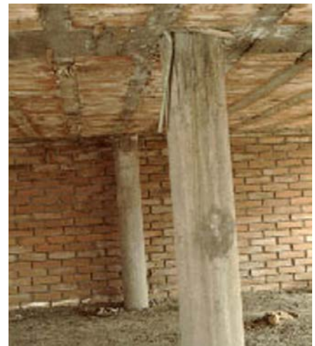
Figure 5A: Poor Construction Practices: Beams constructed in one direction only
