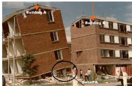
Figure 6E: Collapsed building: Detail A shows too widely spaced stirrups
