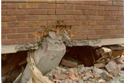
Figure 6D: Earthquake Damage: Inadequate longitudinal and transverse reinforcement (Note the collapsed first story)
