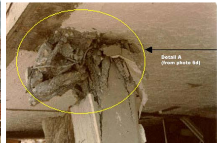
Figure 6F: Collapsed building: Detail A shows too widely spaced stirrups
