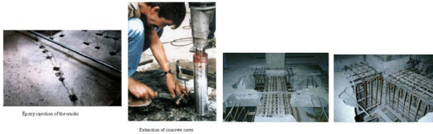
Figure 7D: Seismic Strengthening Techniques: Field Implementation
