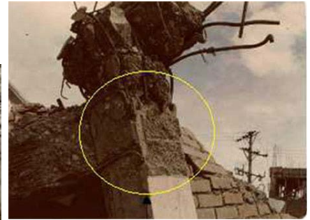
Figure 6C: Earthquake Damage: Anchorage of beam reinforcement in the column cover area (It would be correct to anchor the reinforcement inside the joint.) Detail B
