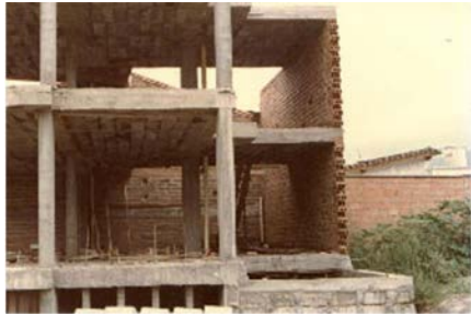
Figure 5E: Poor Design: Combination of Concrete Frames and Unreinforced Masonry Walls or Pilasters
