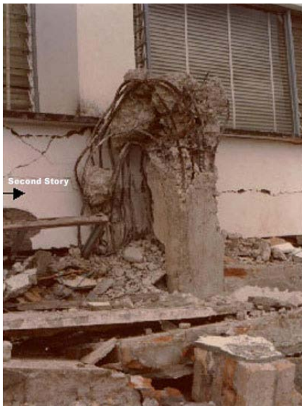
Figure 6G: Collapsed 3-story building. (Note the total lateral drift between the 2nd and 3rd floor.)
