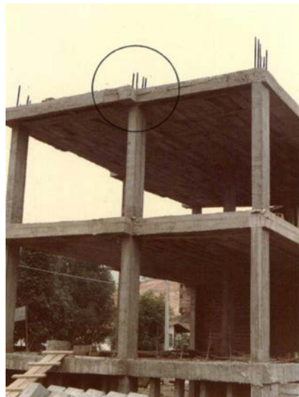
Figure 5C: Poor Construction Practice: Inadequate splice length and location (100% splices at the column base)
