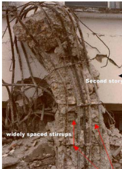
Figure 6H: First-story column collapse due to the widely spaced stirrups and poor quality of aggregate
