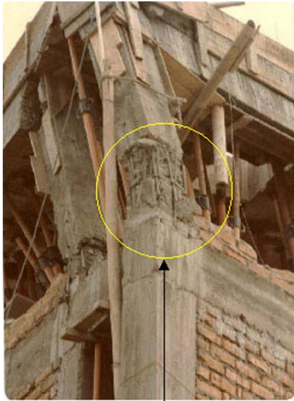
Figure 6J: Earthquake Damage: Inadequate Columns Splices
