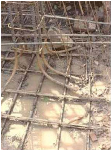
Figure 5H: Poor Workmanship: Dirty groundwork and inappropriate column and beams
