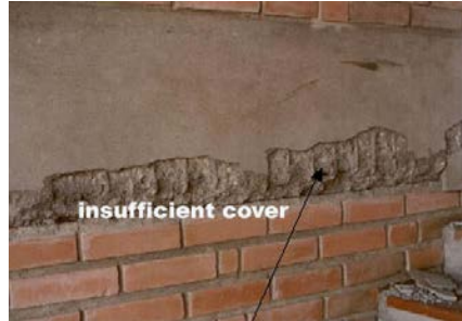
Figure 6K: Earthquake Damage: Inadequate Concrete Cover
