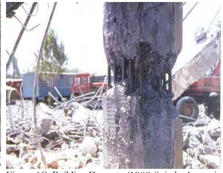
Figure 6C: Building Damage (1988 Spitak, Armenia Earthquake)
