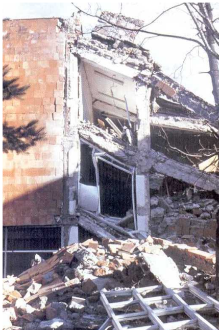
Figure 6D: Building Damage (1988 Spitak, Armenia Earthquake) Source: Klyachko 1999
