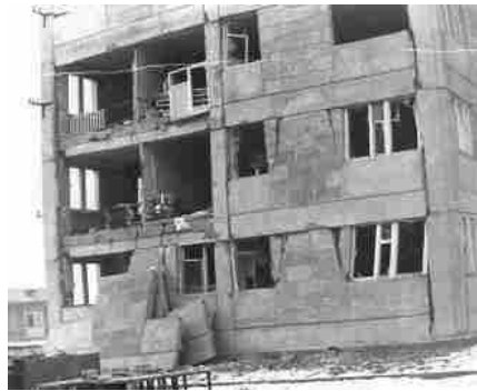
Figure 6B: Building Damage in Leninakan (1988 Spitak, Armenia Earthquake)
