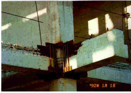
Figure 7A: Illustration of Seismic Strengthening Techniques
