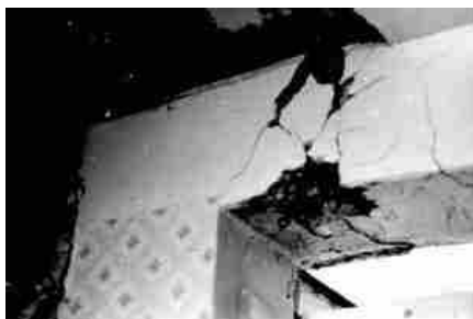
Figure 6A: Building Damage in Leninakan (1988)
