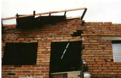
Figure 5E: Key Seismic Deficiencies: Discontinuous Boundary Members
