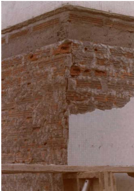
Figure 7D: Seismic-strengthening Techniques: Construction of the Wall-Roof Connection
