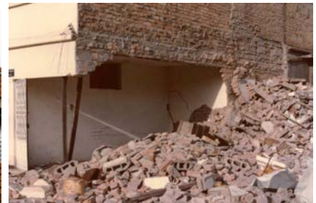
Figure 6: Typical Earthquake Damage: Partial Collapse
