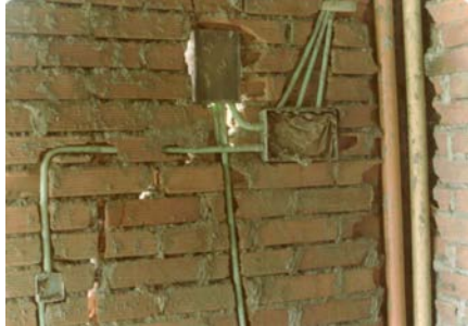
Figure 5A: Key Seismic Deficiencies: Wall Weakness due to Electrical and Water Conduits
