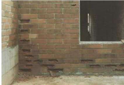
Figure 5B: Key Seismic Deficiencies: Poor Quality of Materials
