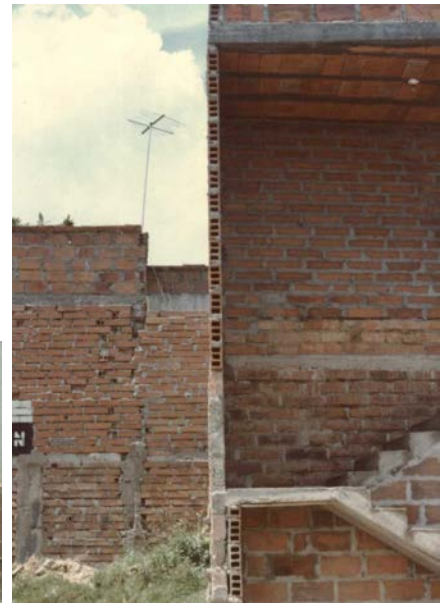
Figure 5C: Key Seismic Deficiencies: Very Slender Walls
