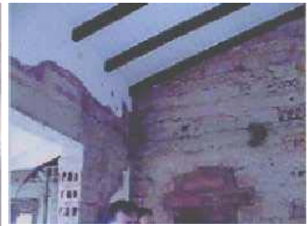
Figure 7C: Seismic-strengthening Techniques: Construction of New Bond Beams
