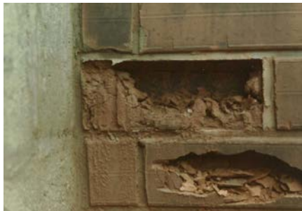
Figure 5D: Key Seismic Deficiencies: Poor Quality of Materials
