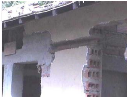
Figure 7B: Seismic-strengthening Techniques: Construction of New Columns and Bond Beams
