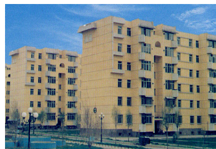
Figure 6B: Base Isolated Brick Masonry Building Undamaged in the 1996 Yunan Earthquake (Magnitude 7.0)
