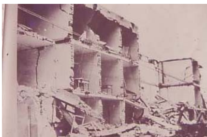
Figure 6A: Typical Earthquake Damage of Brick Masonry Buildings Without Base Isolation (1976 Tangshan Earthquake)
