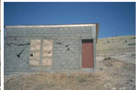
Figure 6C: Earthquake damage (1997 Punitaqui earthquake)
