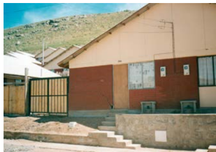
Figure 6B: Earthquake damage (1997 Punitaqui earthquake)
