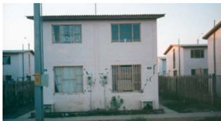
Figure 6A: Photograph illustrating typical earthquake damage (1997 Punitaqui earthquake)
