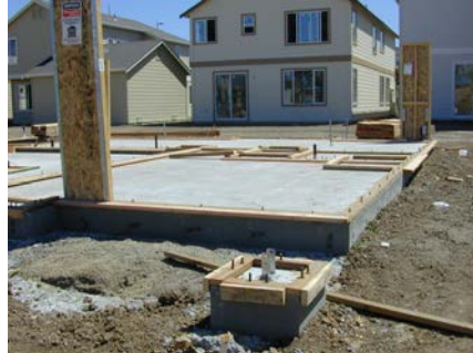
Figure 4B: Some wall framing is now installed
