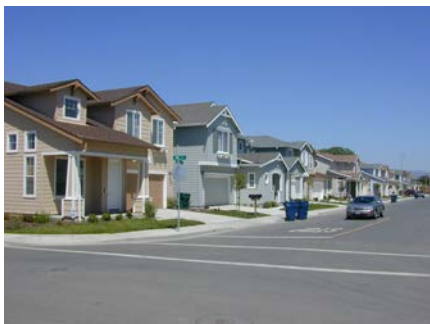
Figure 1A: Typical Building
