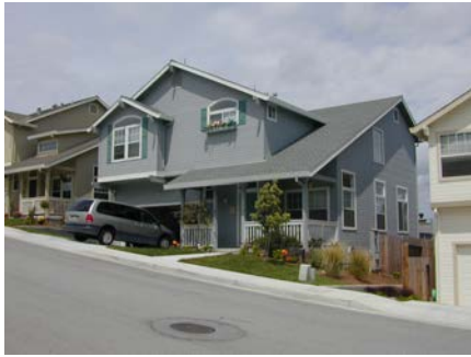
Figure 1D: Partial one and two-story house on sloping site
