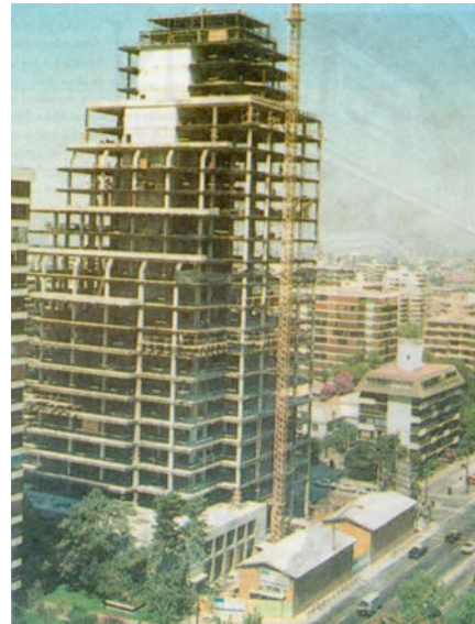
Figure 1B: Typical building
