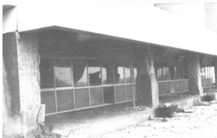
Figure 6D: Medicine School, University of Valparaiso, 1985 Llolleo earthquake, damage in
