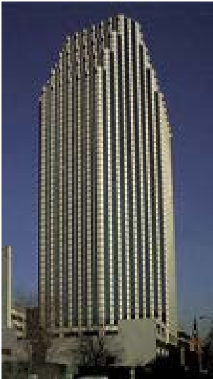
Figure 1A: Typical building
