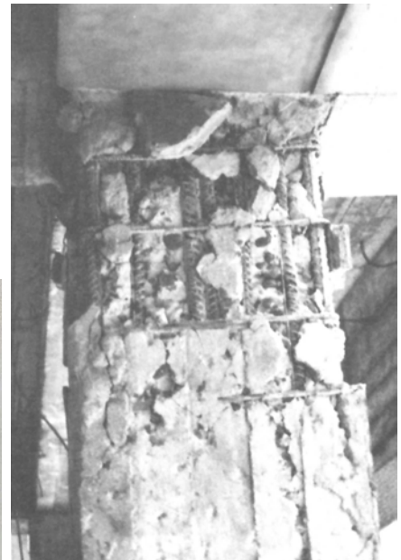
Figure 6C: San Antonio Hospital, close-up damaged in the 1985 Llolleo earthquake
