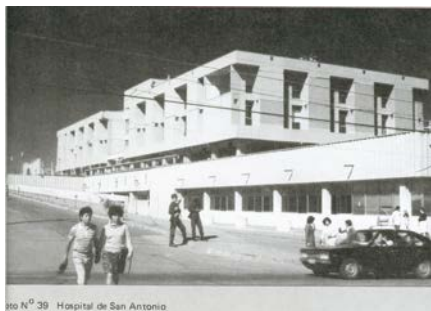
Figure 6A: San Antonio Hospital, March 3, 1985 Llolleo earthquake
