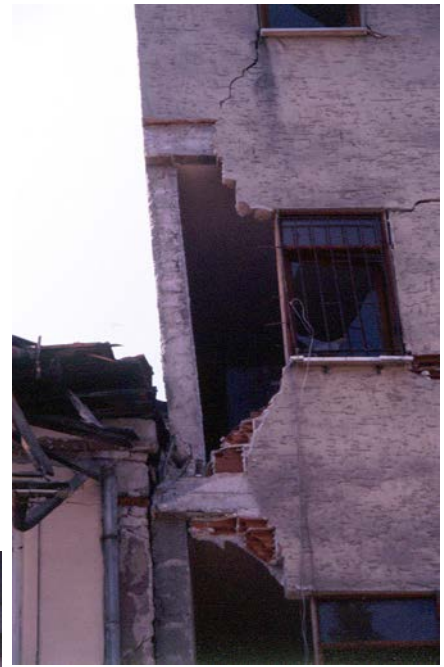
Figure 6L: Typical Earthquake Damage - Pounding Between a Six-Story Building and a Two-Story Building in Golcuk, Causing Damage to the Column of th Six-Story Building (EERI 2000)
