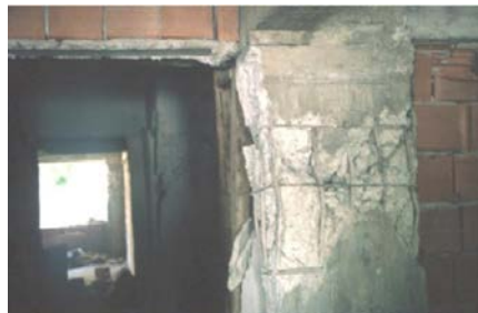
Figure 6H: Typical Earthquake Damage - Column Failure
