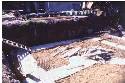
Figure 4B: Critical Structural Details - Heavy Mat Slab Foundation (EERI 2000)
