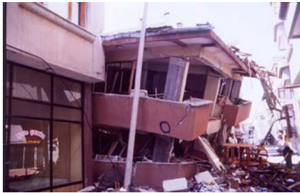
Figure 6D: Typical Earthquake Damage - Pullout of Column Reinforcement in a Low-Rise Building in Adapazari (EERI 2000)
