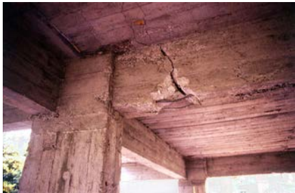
Figure 6M: Typical Earthquake Damage Due to Pounding Effect (detail of a six-story building shown on the previous figure) (EERI 2000)
