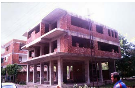
Figure 4A: Critical Structural Details - Irregular Column Orientations and Layout (EERI 2000)
