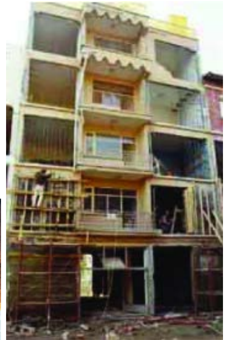
Figure 6O: Typical Earthquake Damage to a Building Under Construction, Revealing Eccentric Beam-Column Framing, Beam Longitudinal Bars Located Outside the Column Cage, and Infrequent Transverse Hoops (EERI 2000)
