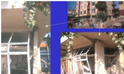
Figure 6G: Typical Earthquake Damage: Weak-Story Mechanism Developed in the Bottom Story
