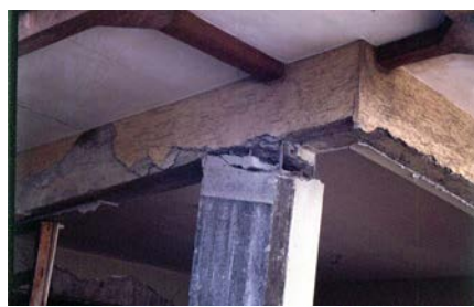
Figure 6E: Typical Earthquake Damage - Close Up of Uppermost Corner Column Joint in the Building Shown on the Previous Figure (EERI 2000)
