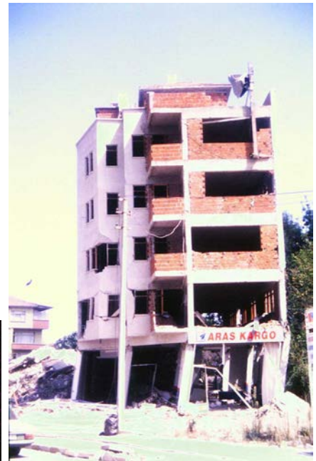
Figure 5: Key Seismic Deficiencies - A Weak-Story Mechanism Developed at the First Floor (the case of the lowest floor used for commercial purposes and lacking the stiffness provided by the infill at the upper floors (EERI 2000)
