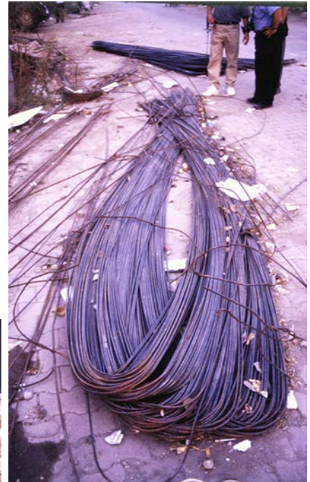
Figure 4C: Critical Structural Details - Smooth Reinforcing Steel Delivered to a Construction Site Bent into a "U" Shape (no material certification provided) (EERI 2000)
