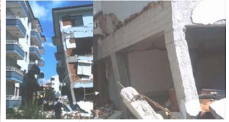
Figure 6C: Typical Earthquake Damage
