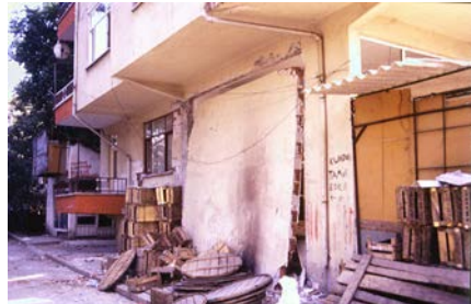
Figure 6B: Typical Earthquake Damage - Hollow Clay Tile Wall "popped" out from a Six-Story Building in Golcuk (EERI 2000)
