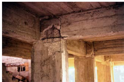
Figure 6N: Typical Earthquake Damage - Building Under Construction, Revealing Location of Central Bent-Up Longitudinal Beam Bar, Infrequent Stirrups, and Beams Framing Eccentrically Into Columns (EERI 2000)
