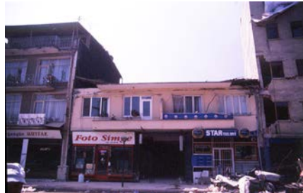
Figure 6K: Typical Earthquake Damage to Beam-Column Joints of an Irregular building in Adapazari Maintaining Gravity Load Support (EERI 2000)
