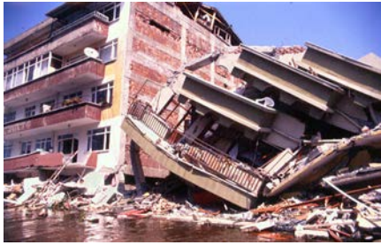
Figure 6A: Typical Earthquake Damage - Multiple-Story Collapse in a Six-story building at Golcuk (EERI 2000)
