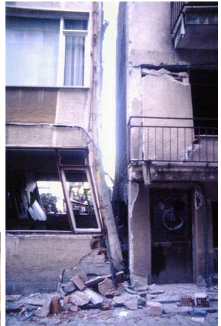
Figure 6F: Typical Earthquake Damage: Weak-story Mechanism Developed in the Building at the left (note columns oriented to increase the glazing area). The columns at the front of the building at the right are oriented perpendicular to those of the building.
