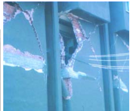
Figure 6I: Typical Earthquake Damage - Pier Failure
