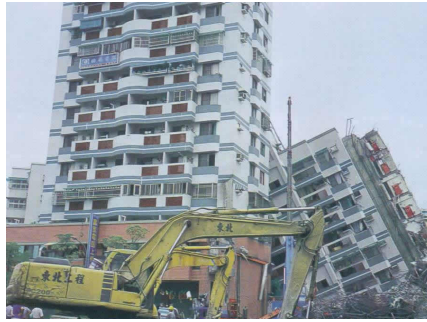
Figure 5: A Photograph Illustrating Typical Earthquake Damage
