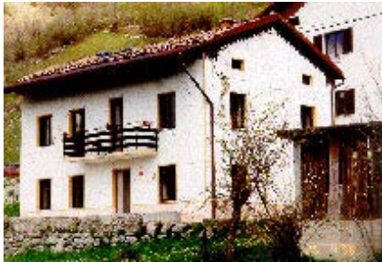
Figure 1A: Typical Building
