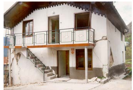
Figure 5A: an Illustration of Key Seismic Deficiencies - lack of structural integrity results in wall dislocation and corner damage
