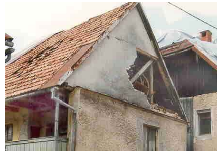
Figure 6B: Out-of-plane gable collapse
