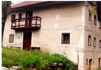
Figure 7E: A building strengthened after the 1976 Friuli earthquake remained undamaged in the 1998 Bovec earthquake
