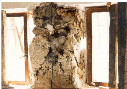
Figure 5B: Seismic deficiency: pier failure
