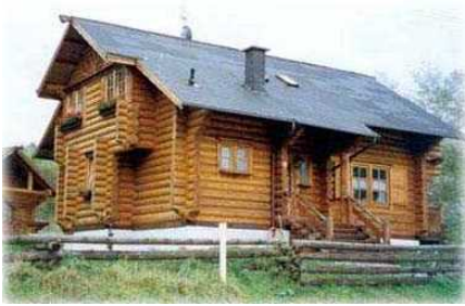
Figure 1A: Typical Building
