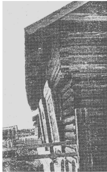
Figure 5B: Wall damage in the 1958 Kamchatka earthquake (showing a side view of the building)
