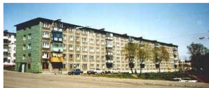
Figure 1B: Typical Building on Seria 135
