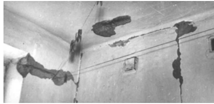
Figure 5E: Typical Earthquake damage - Interior View of Damages
