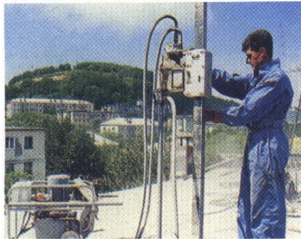
Figure 6B: Seismic Strengthening: Application of Post-Tensioning System
