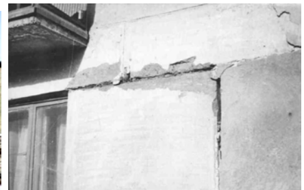
Figure 5C: Typical Earthquake Damage- Shearing of Blocks at the Joint Locations
