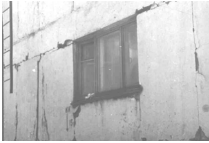
Figure 5D: Typical Earthquake Damage- Shearing of Blocks at the Ground Floor Level
