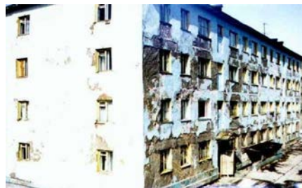
Figure 5B: Typical Earthquake Damage - A View of the Damaged Building
