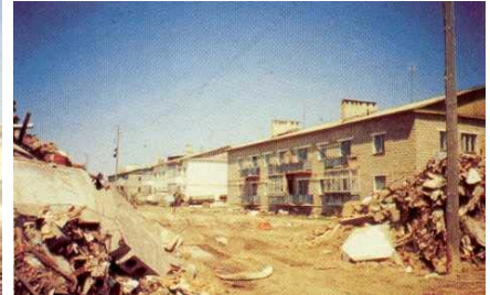
Figure 5I: Two-Story Large-Block Masonry Buildings Did Not Suffer Major Damage in the 1995 Neftegorsk Earthquake (Source: Klyachko, 1999)
