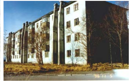
Figure 6C: A building Strengthened using Post-Tensioning System
