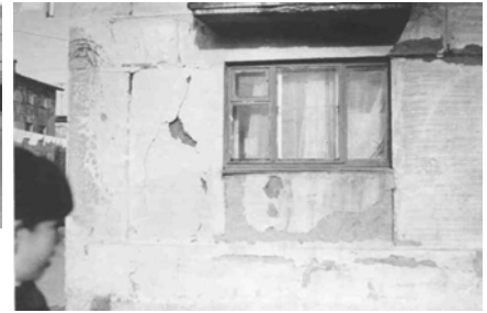
Figure 5F: Typical Earthquake Damage at the Wall Corner
