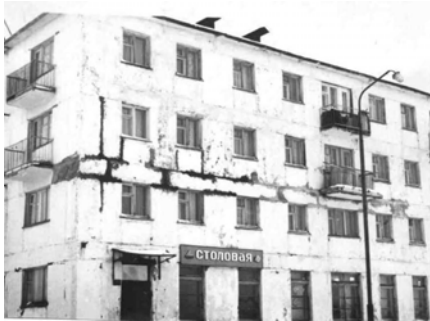
Figure 5G: Typical Earthquake Damage- Shearing Failure of Blocks at the Joint Locations
