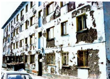
Figure 5A: Typical Earthquake Damage to the exterior longitudinal walls
