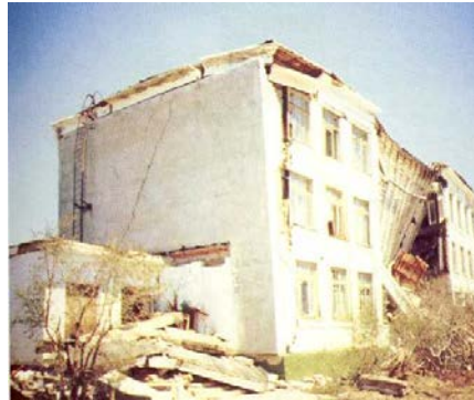
Figure 5H: Collapse of Five-Story Large-Block Masonry Buildings (1995 Neftegorsk earthquake)- Source: Klyachko (1999)
