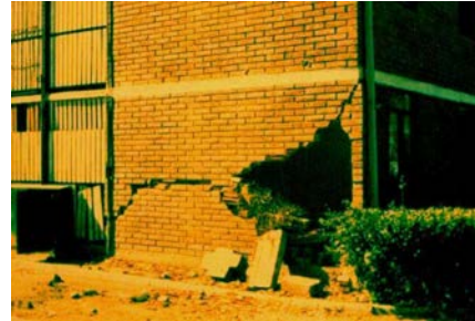
Figure 6B: Failure of masonry walls in March 3, 1985 Lolleo earthquake
