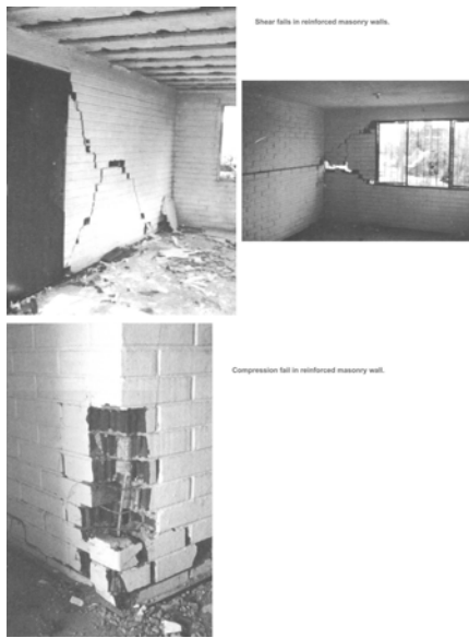
Figure 6A: March 3, 1985 earthquake in Central Chile. Damage to masonry buildings in Santiago.
