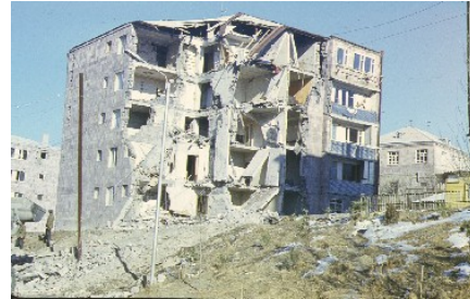
Figure 5A: A Photograph Illustrating Typical Earthquake Damage (Spitak, Armenia earthquake 1988)
