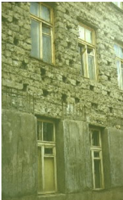
Figure 6E: A Building Strengthening Using the Method of Added Stiffness
