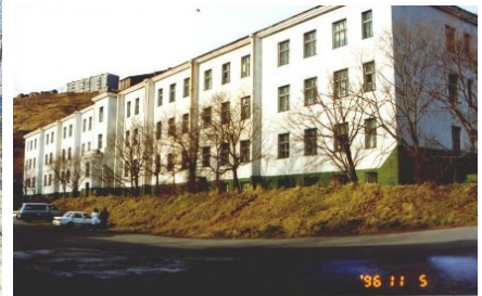
Figure 6C: A building Strengthened using Post-Tensioning System
