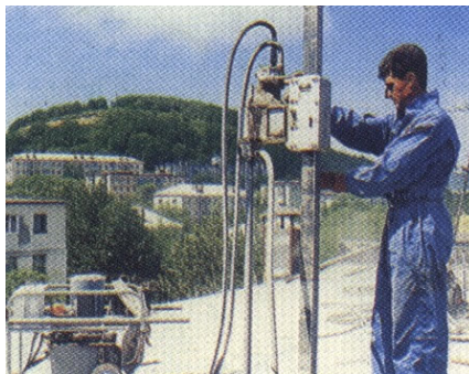
Figure 6B: Seismic Strengthening: Application of Post-Tensioning System
