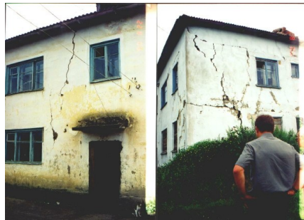
Figure 5B: Typical Earthquake Damage
