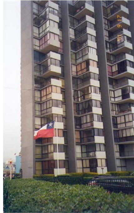
Figure 7B: Seismic strengthening (Edificio Acapulco building). The exterior wall has been thickened with a new steel mesh.
