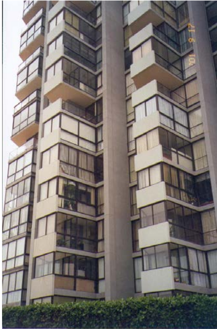
Figure 7A: Seismic strengthening (Edificio Acapulco building damaged in the 1985 Lolleo earthquake). A column has been added to the wall exterior.
