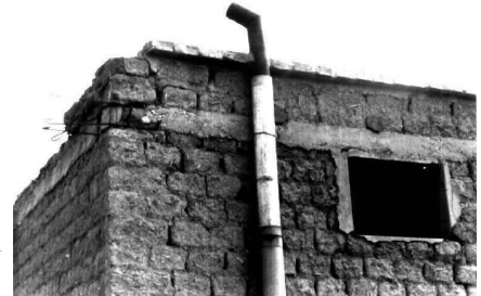
Figure 7: Photograph illustrating typical earthquake damage
