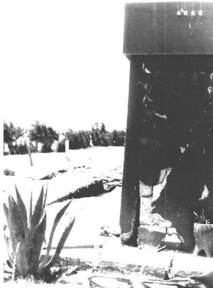
Figure 5: Photograph illustrating typical earthquake damage
