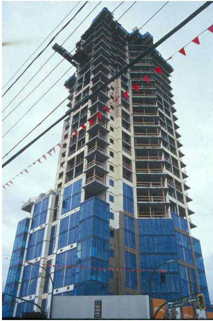
A Typical Building Under Construction
